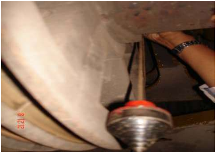
Figure 3.5. Checking the verticality of Axle pulley
