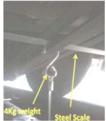
Figure 2.8. Checking of V belt tension with 4 kg weight and steel scale
