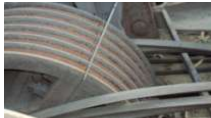
Figure 2.6. Checking of gap between two halves of Axle pulley
