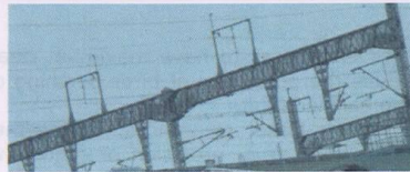
JAPAN RAILWAY-NYLON NET ON PORTAL BOOM & DROP ARM
