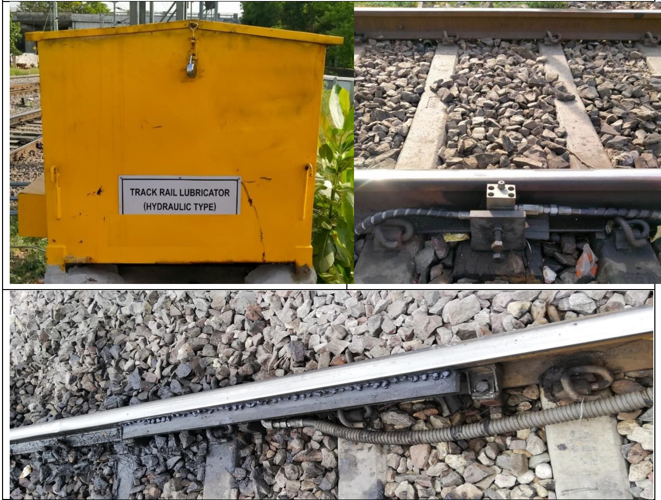
Track Based lubricator (Hydraulic Type )
