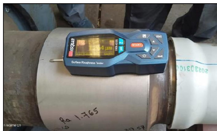
Surface roughness checking
