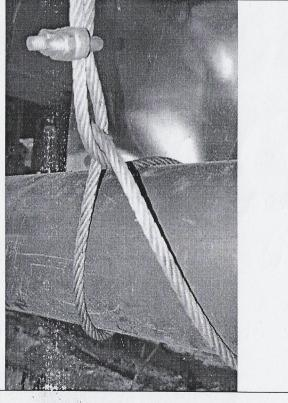
3 Secure the free end of safety sling with help of U-clamp (bull dog clamps).
