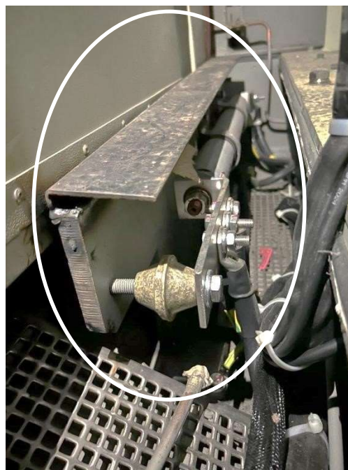
Fig-4: After removal of FB Cubicle
