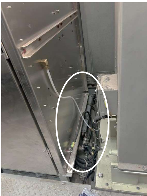
Fig-3: Before removal of FB Cubicle
