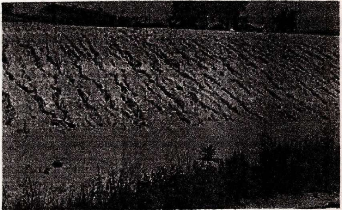
Erosion in Slopes
