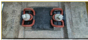
Fig- 4 : Fastening Assembly on Booted Block
