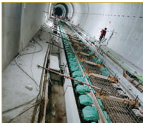
Fig. 31: Covering Block with polythene
