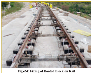
Fig-24: Fixing of Booted Block on Rail
