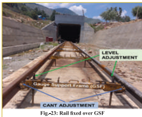
Fig-23: Rail fixed over GSF
