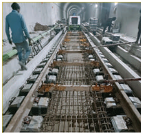
Fig. 25: Reinforcement work completed & turnbuckle anchored from tunnel side
