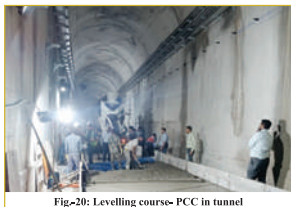
Fig-20: Levelling course- PCC in tunnel
