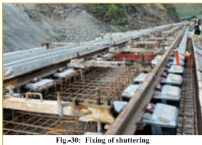
Fig.-30: Fixing of shuttering
