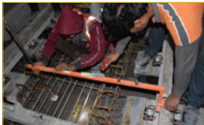
Fig. 27: Alignment with Center Gauge
