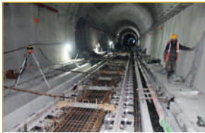
Fig. 28: Rail level checking with digital level
