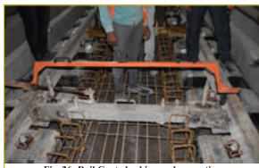
Fig. 26: Rail Cant checking and correction
