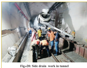
Fig-20: Side drain work in tunnel
