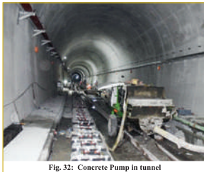
Fig. 32: Concrete Pump in tunnel
