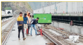
Fig-22: Lifting of Rail and supporting on wooden block
