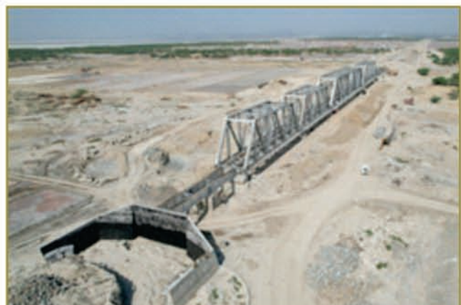
Construction of Bridge
