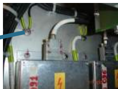
Ground termination of ALG Rack connected with the DC Link voltage sensor ground
