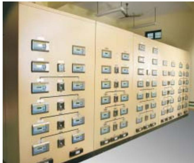
**Fig. 5 : Control and relay panel for TSS**
